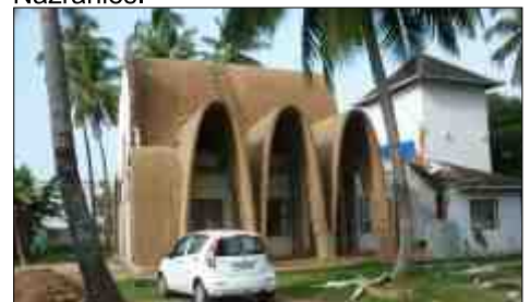
Church renovation progress as on 27 Oct 2012
