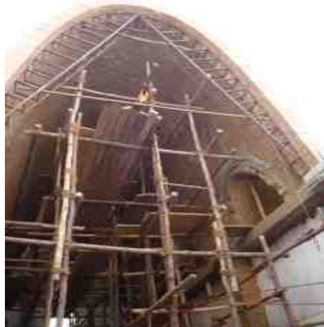
Vaults under construction
