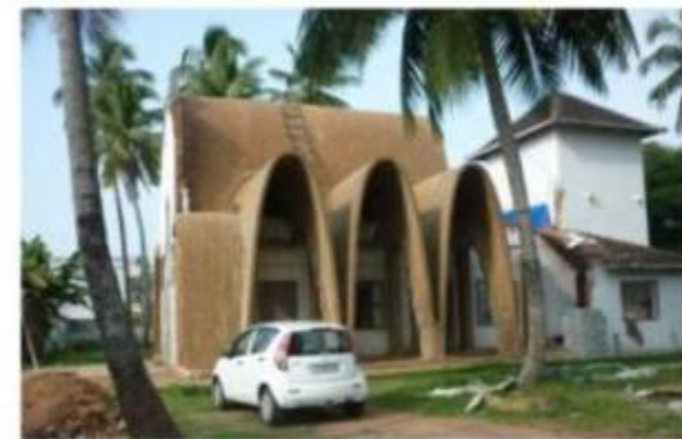
Church renovation progress as on 27 Oct 2012
