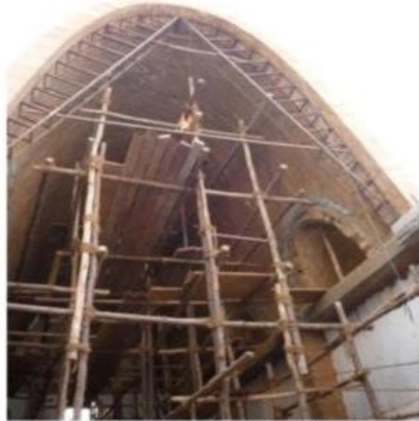
Vaults under construction
