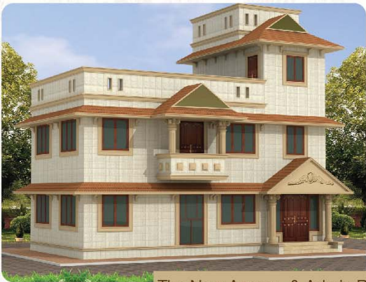
The New Accom. & Admin Block
